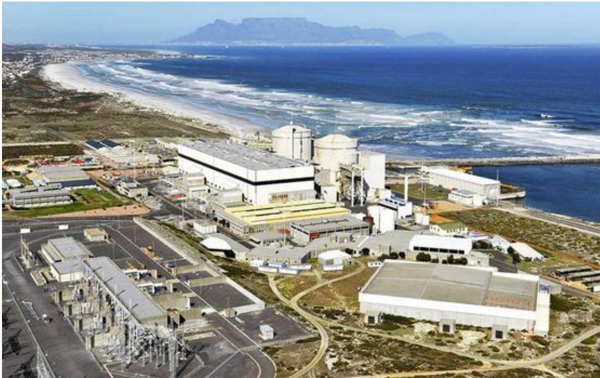
Koeberg Power Station
